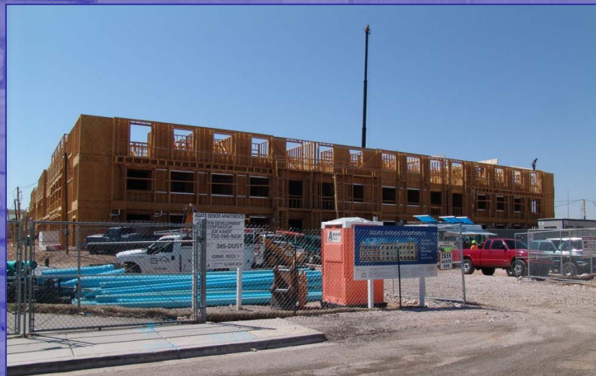
Accessible Space, Inc. Agate Avenue Senior Apartments under construction
